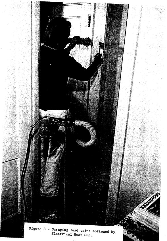
generally observed that the ease of stripping increased with increasing paint thickness probably because of the greater absorption and retention of heat and the greater entrapment of solvents in the old coatings.
